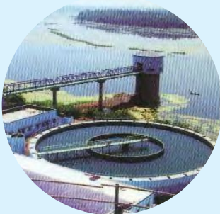
Water Treatment Plant
